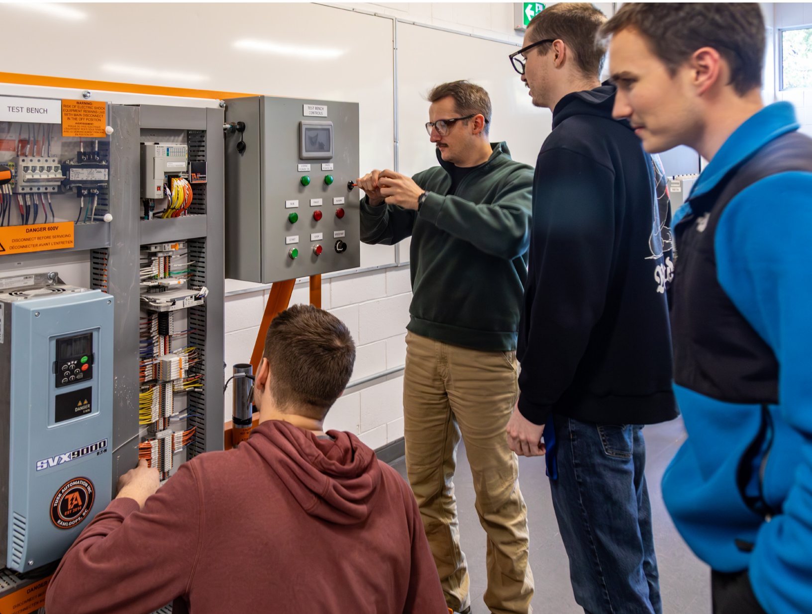
In 2025, Coast Mountain College received the donation of an electrical test bench from Brucejack Mine, operating under Newmont Canada. The bench will allow students to gain the practical, hands-on skills needed in the electrical trade.
